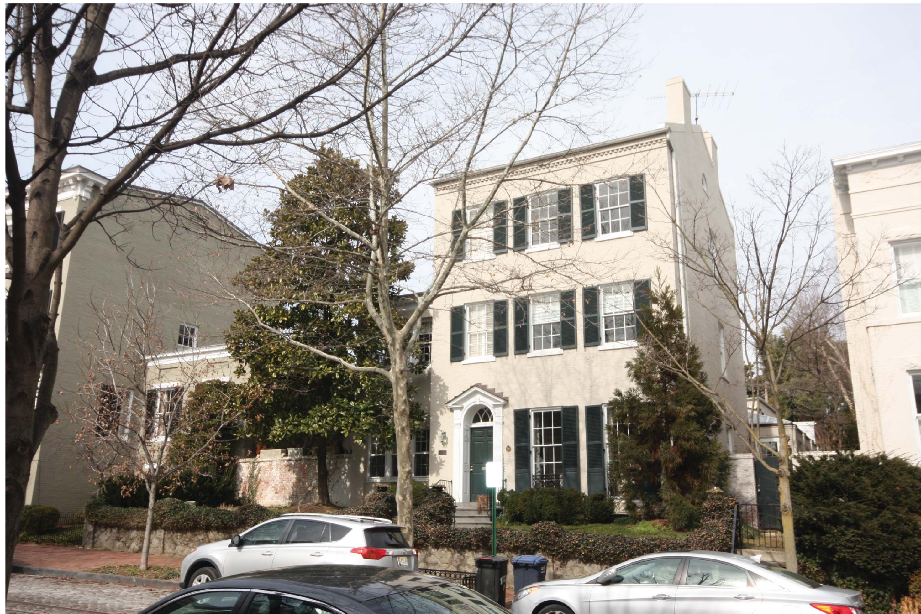
3323 P STREET SOUTH (FRONT) FACADE
