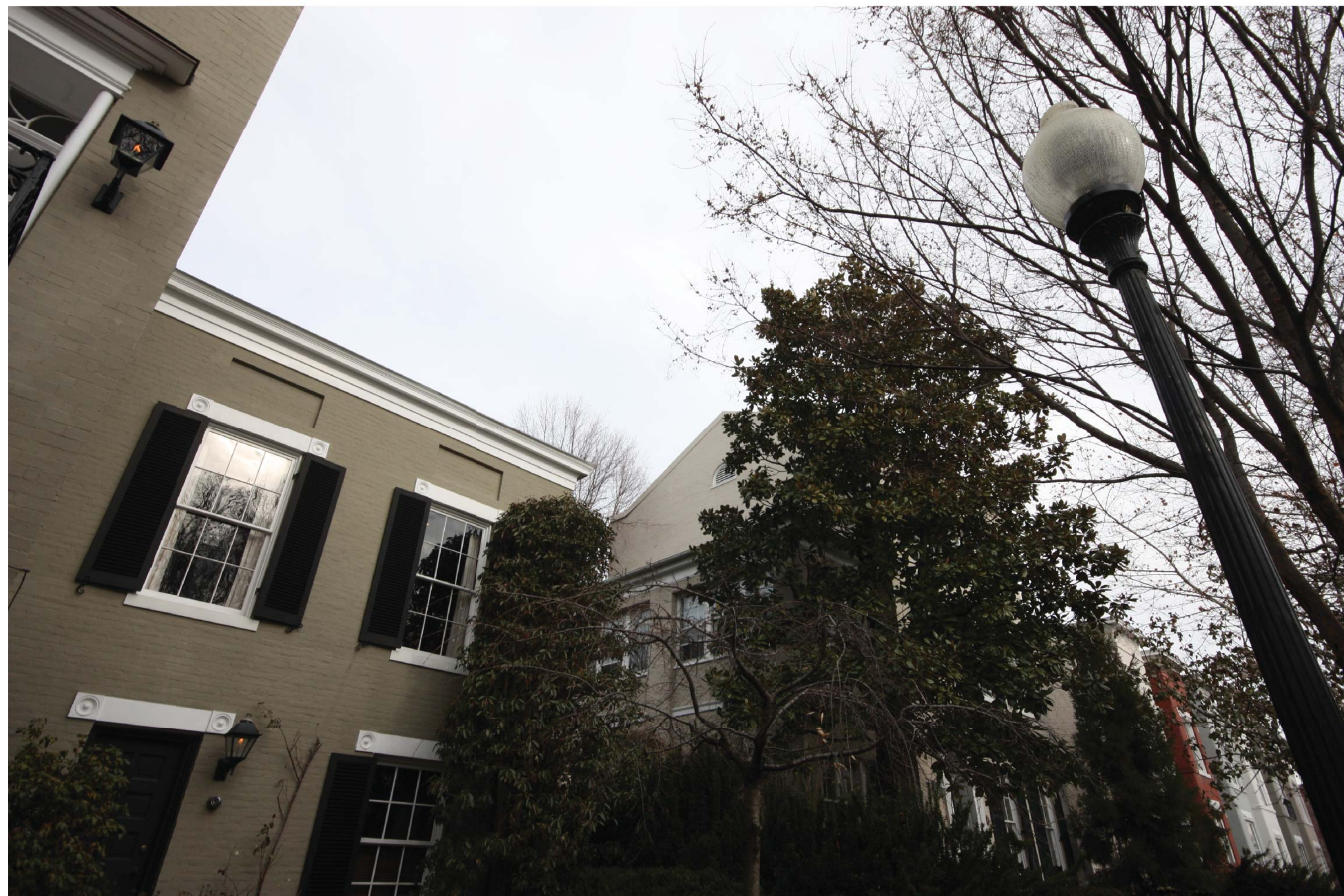
VIEW FROM P STREET (SOUTHWEST)
