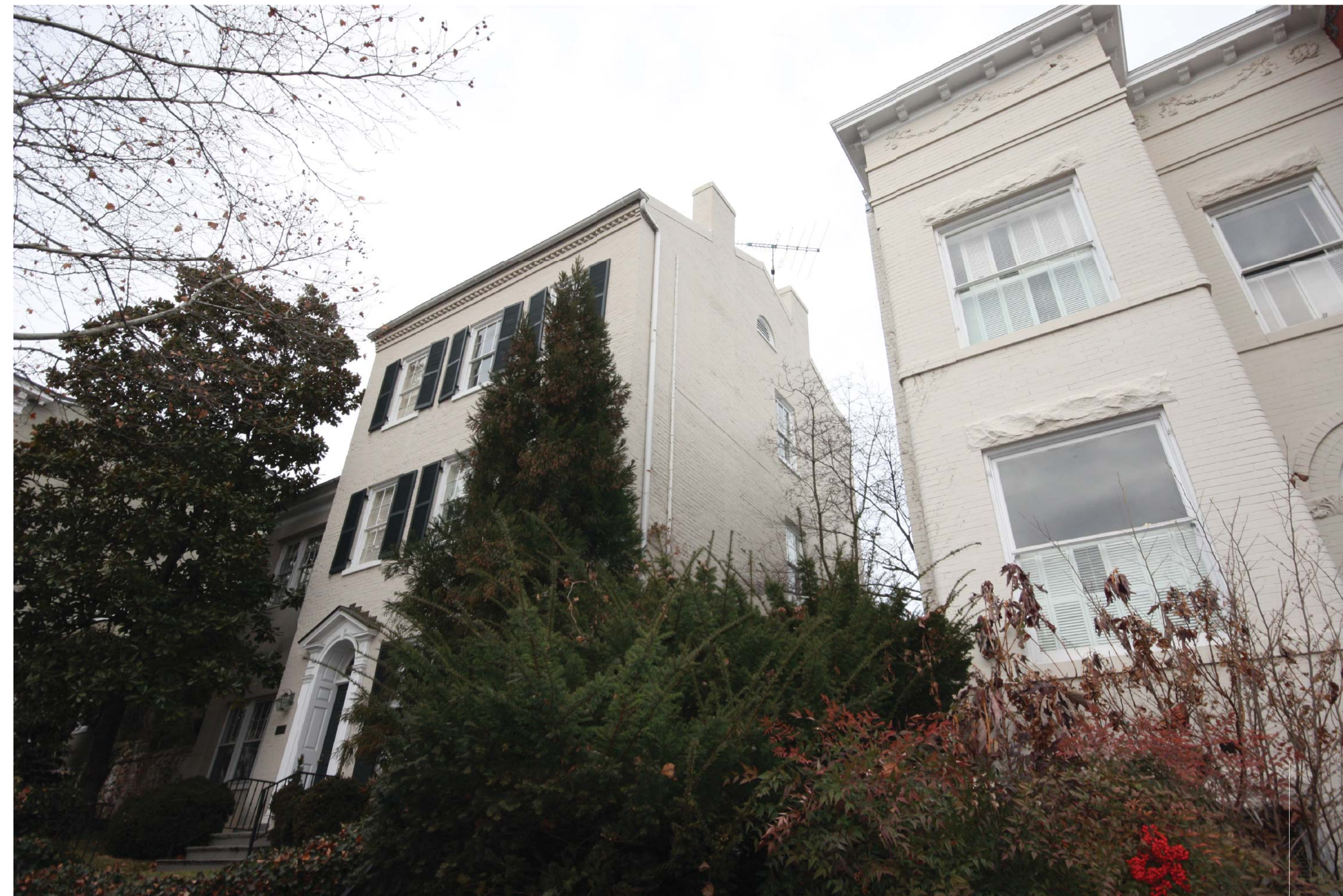
VIEW FROM P STREET (SOUTHEAST)
