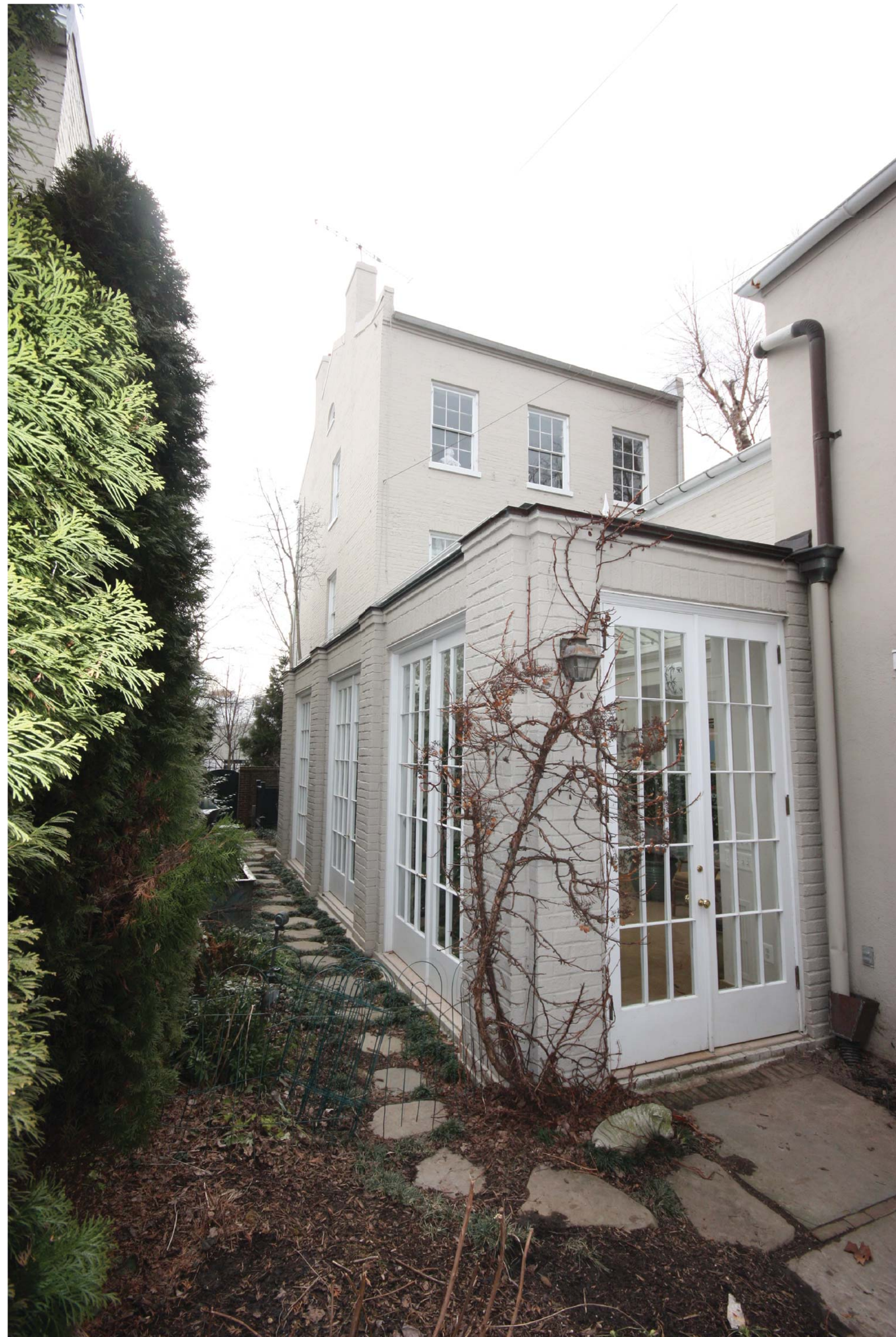
VIEW FROM NORTHEAST (BACK YARD)
