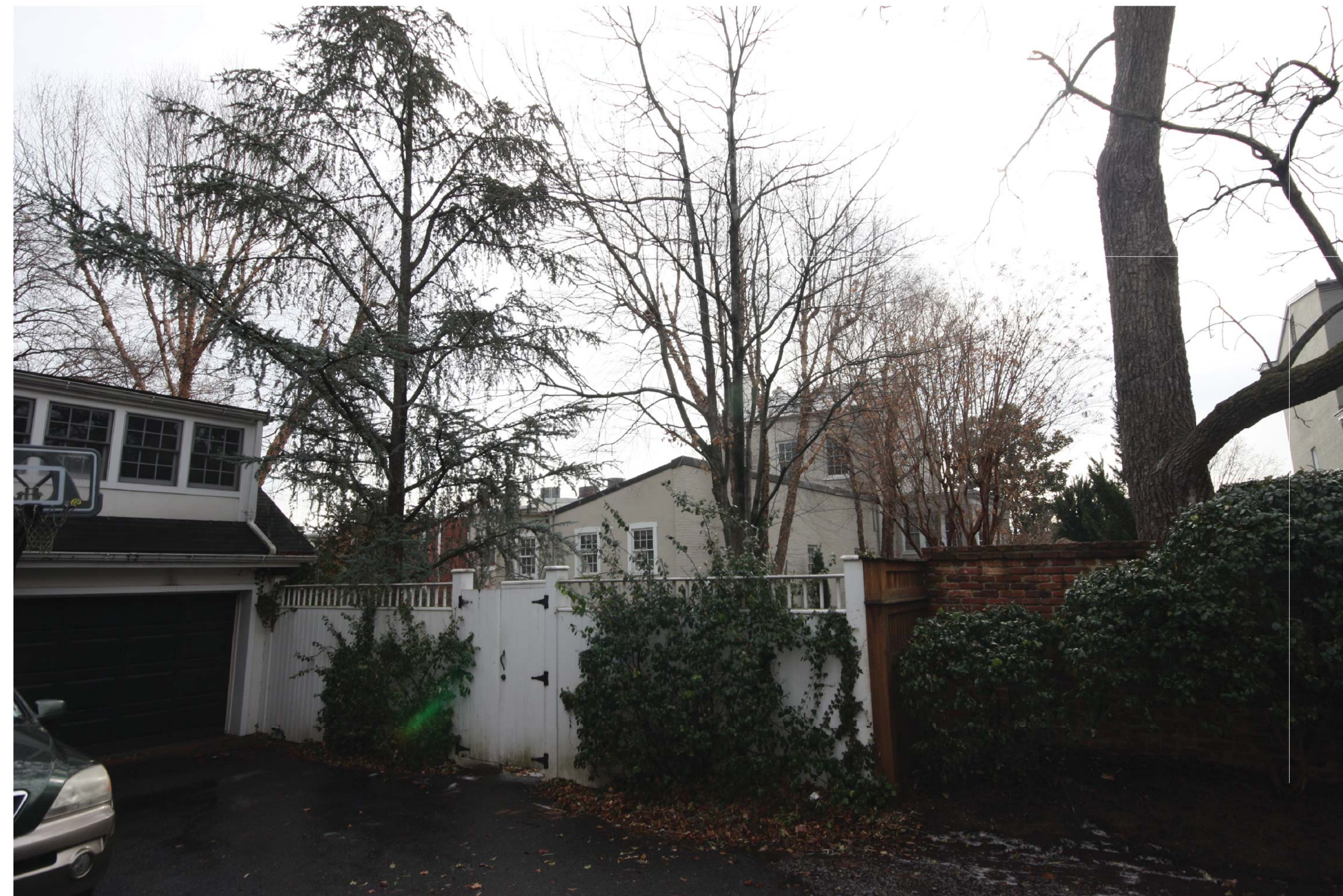
VIEW FROM POMANDER WALK NW (REAR FACADE, NORTH)
